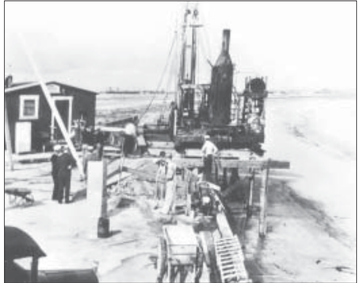
Pile Drivers Building Allen Field—Allen Field was a civilian airfield built in 1927 on Terminal Island, later re-named Reeves Field and used by the Navy during World War II.
